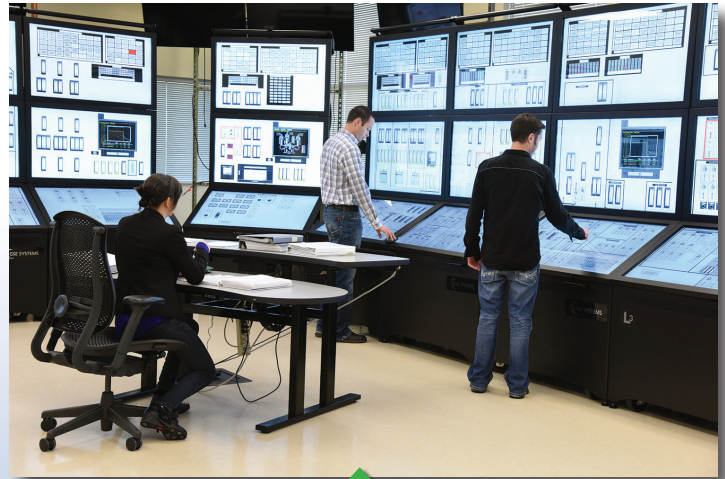
The Human Systems Simulation Laboratory at INL is a reconfigurable virtual control room used for operator training and research.
